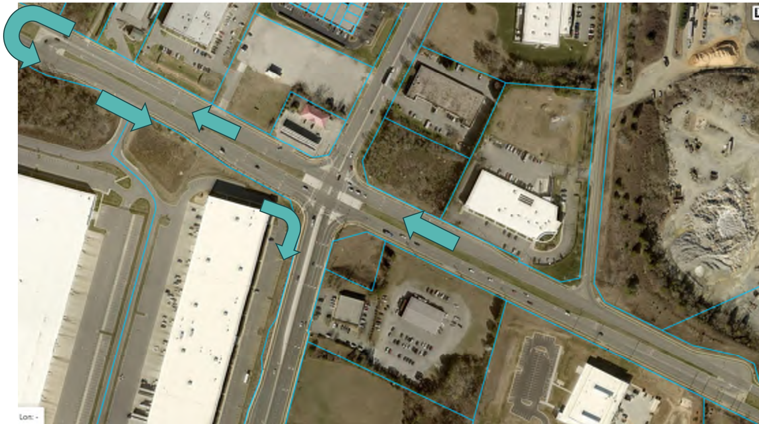
Poplar Tent Rd & Derita Rd, Cabarrus County
